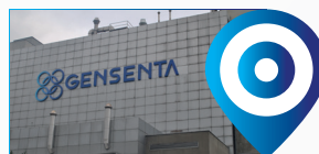
Finished Products Factory, Istanbul
